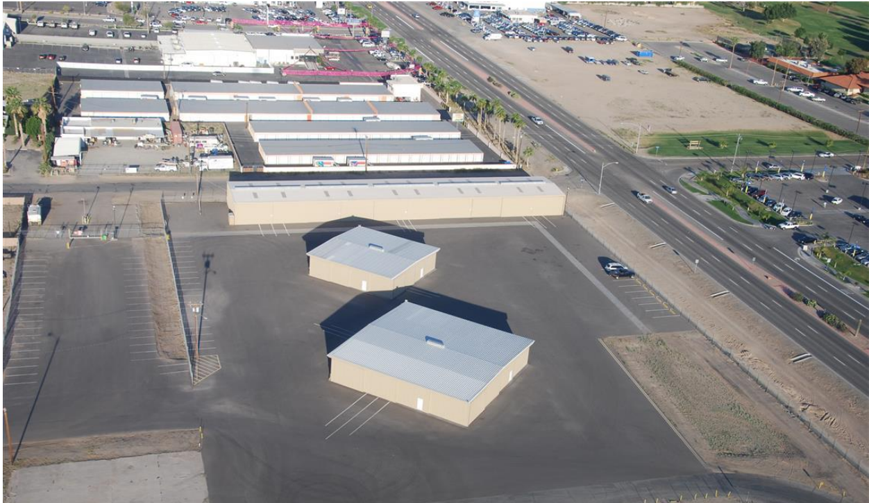
Figure 1-16: Northwest GA Hangars
