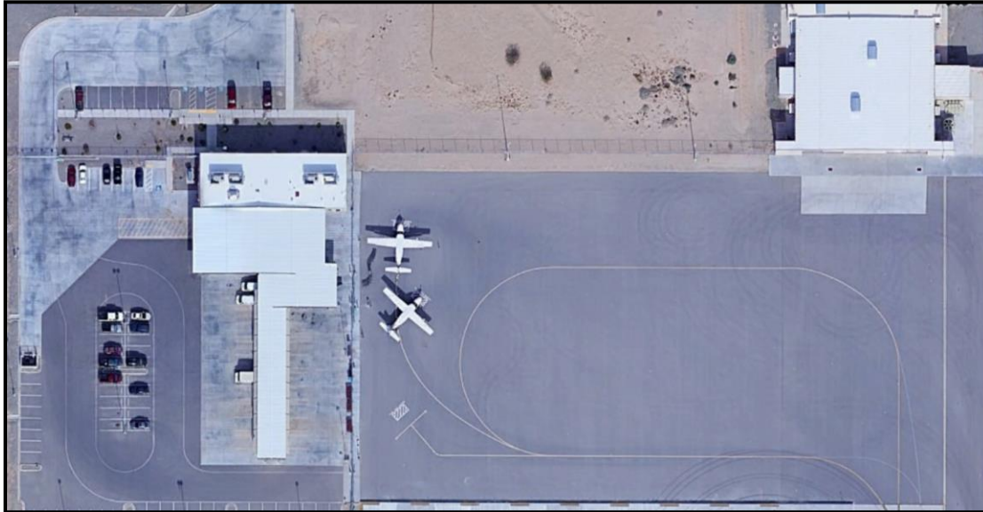
Figure 4-21: Air Cargo Apron Facilities
